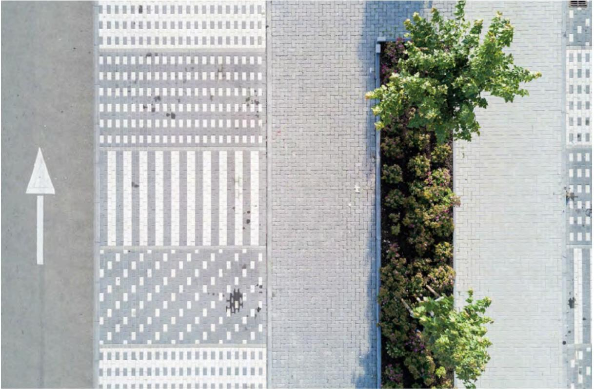
*Figure 4.8: Image from Smart Surfaces Guide: Example of Asphalt with High Solar Reflective and Permeable Surfaces. The additional incorporation of Bioswales help reduce Urban Heat Island and increase natural Stormwater infiltration.*
