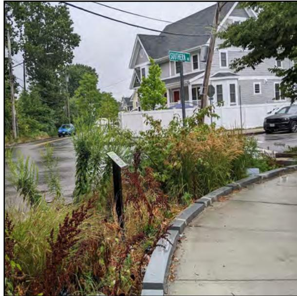
Figure 4.11: New England Avenue Bioretention. (photo: City of Boston)
